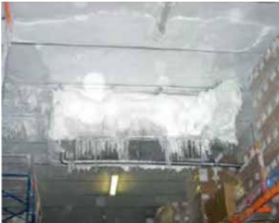
Poor control of doors and of defrosting in a cold store – a dangerous combination. This evaporator is completely iced up, meaning that it will be providing a fraction of the necessary cooling, but with increased energy consumption.
