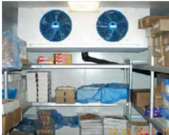
A freezer room with a nicely defrosted evaporator and a well insulated drain – as well as low-power fans. No evidence of ice.
